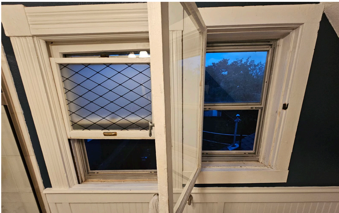
Photo 2: Upstairs Bathroom double-hung window and casement window
